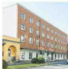
Urban center in corso Cavour
